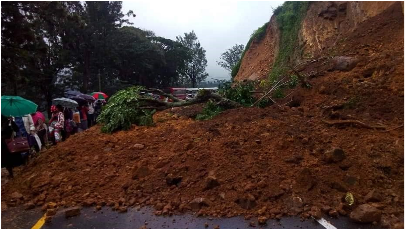
FIGURE 05: Road block due to earth slip in Badulla
