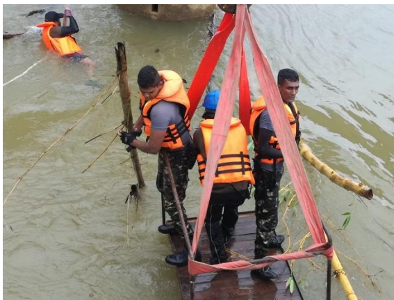
(Debris Cleaning in Weliwita Divithura bridge)
